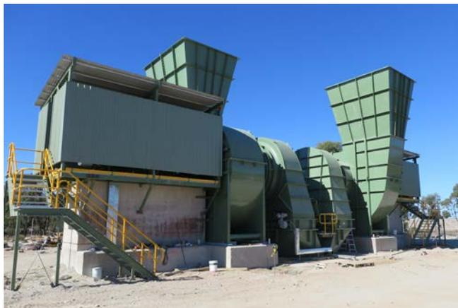
Figure 2: Ventilation Fans installed at Tritton Underground Mine over the new exhaust ventilation shaft
